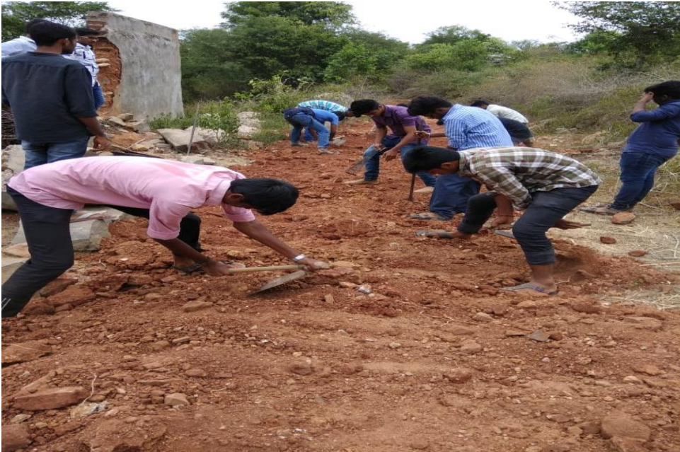
Day – 3 Road leveling works
